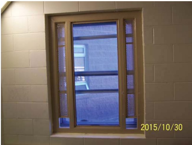
Port-Cartier Institution Segregation Cell
